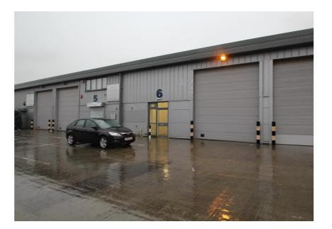
This modern mid terraced, steel framed warehouse/industrial building was constructed in 2007 and provides a clear warehouse area with an eaves height of 5.67 metres (19 feet) rising to 6.68 metres (22 feet) at the apex. The property benefits from fitted first floor offices and WC facilities, as well as good forecourt loading & car parking provision.
